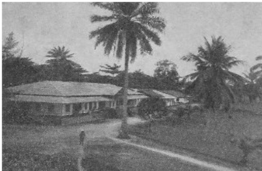
Douala Hospital: "Native Pavilion"
